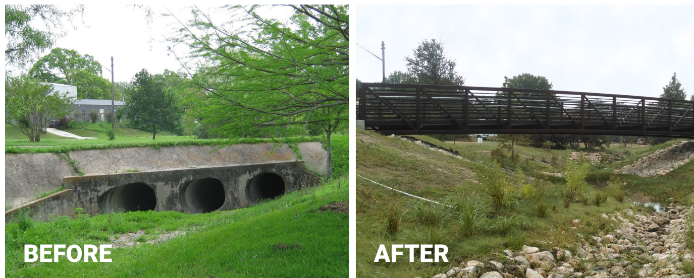
Photos courtesy of City of Austin Watershed Protection Department
