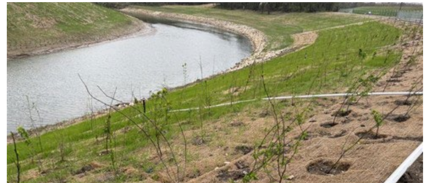
Figure 9.2. Riparian vegetation establishment. This occurred along the West Fork Trinity River in Fort Worth, Texas.
