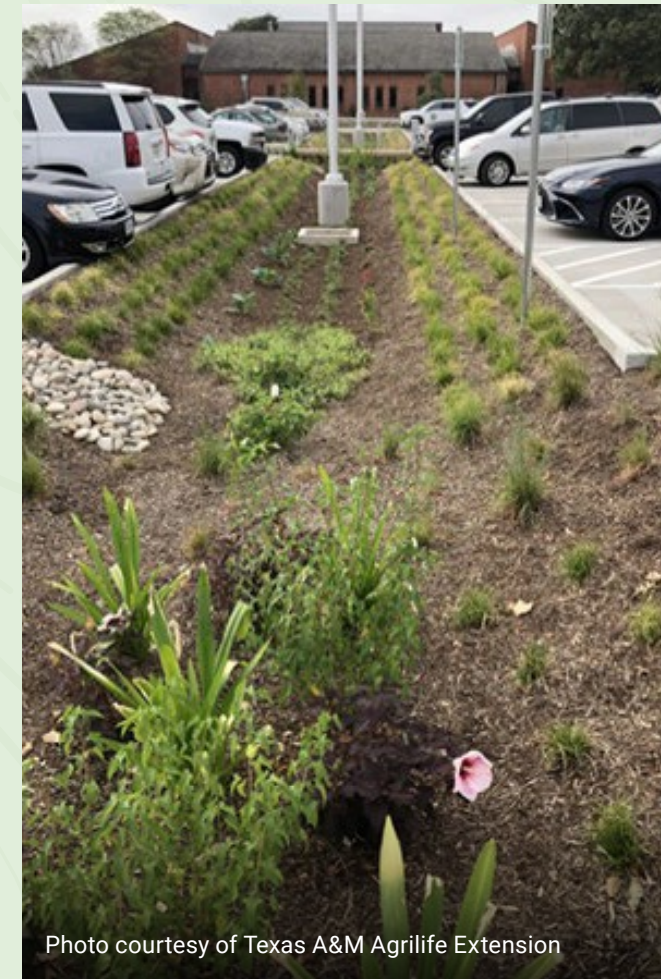
Figure 7-4. Bioretention basin area analyzed near adjacent parking lot
