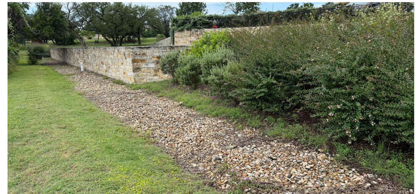
Figure 11-7. Infiltration Trench in Bee Cave, Texas
